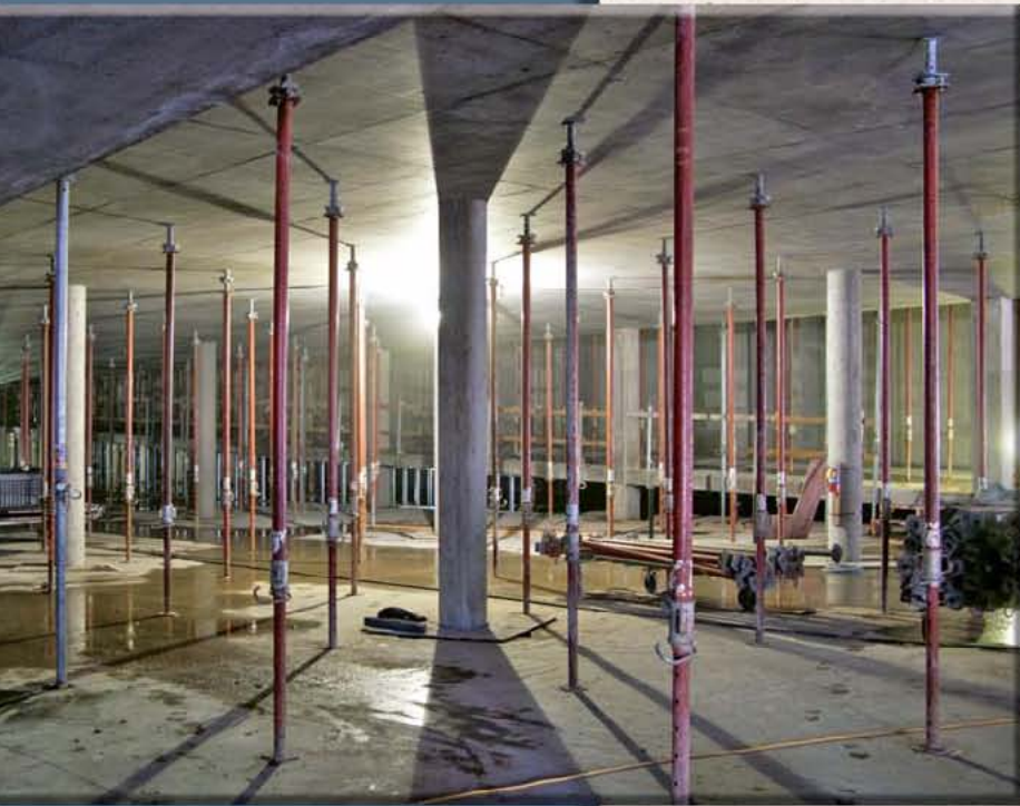
Fresh concrete floor pours are held in place by steel jacks while they dry, as we tour in February. An army of workers is oblivious to midwinter conditions in the Northwest. (Left) A proof-of-concept main roof arch features an incredibly strong glue-lam beam about four feet deep. The site is adjacent to the Tacoma Dome.
