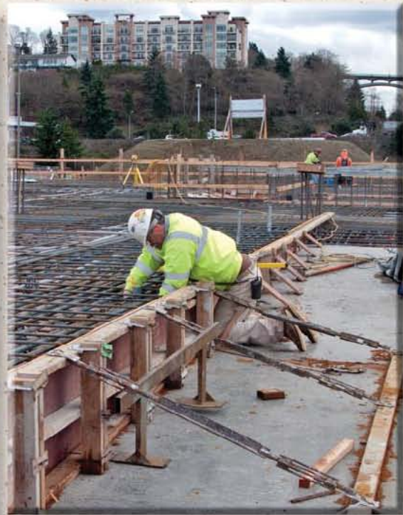
Fresh concrete floor pours are held in place by steel jacks while they dry, as we tour in February. An army of workers is oblivious to midwinter conditions in the Northwest. (Left) A proof-of-concept main roof arch features an incredibly strong glue-lam beam about four feet deep. The site is adjacent to the Tacoma Dome.
